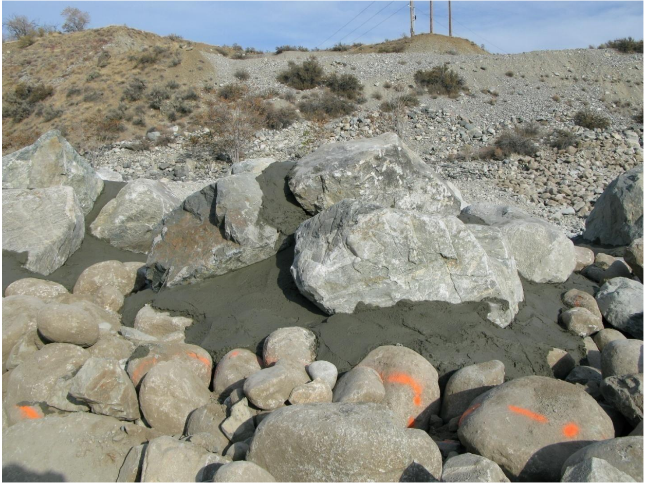
Picture taken on 10/29/08 showing a typical boulder cluster. The newly placed grout locks the boulders together to create a structure that will dissipate energy from flows entering the habitat channel.
