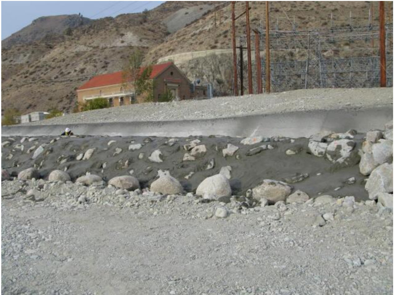
Conveyance canal overflow spillway section under construction, 10/30/08. Boulders have been installed and grout was placed this day.
