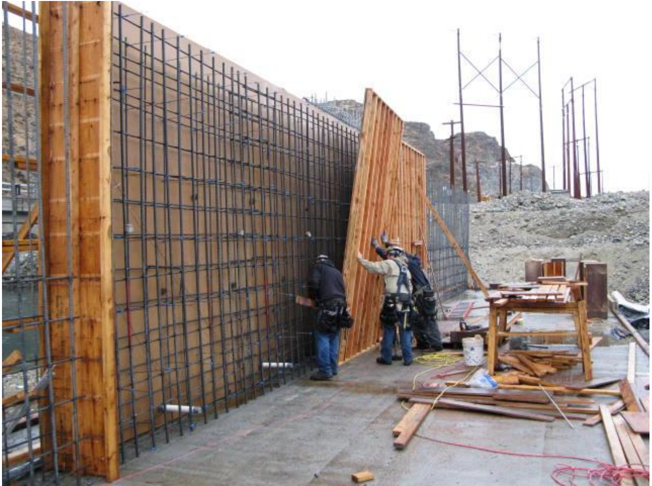
Pump station foundation slab and grade beams have been placed. Retaining wall forms and rebar underway. 11/4/08
