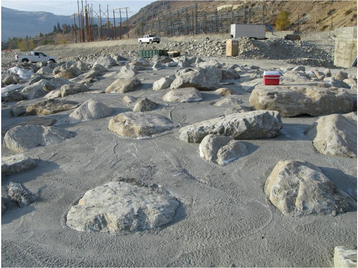
This is the high elevation portion of the hydraulic control structure. Picture taken on 10/29/08, showing previously placed concrete, intended to lock the structure together.
