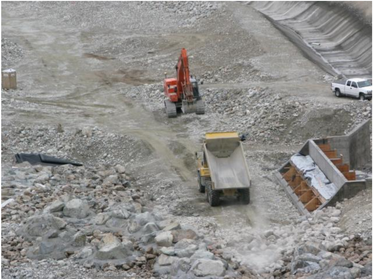
Picture taken on 11/3/08. Concrete for the pumped water outlet structure has been completed, and forms are still in place. Rock embankment material placement is underway.
